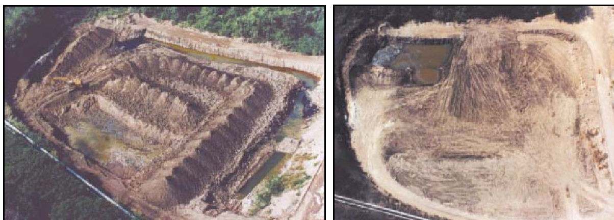
Figures 4+5: During (on the left side) and after (on the right side) the bioremediation of oil base bottom mud with the Intebios® technology in the Pamatacual reserve pits, Puerto La Cruz Refinery, Anzoátegui State, Venezuela in 1997 (duration: 6 months) (INFANTE et al. , 1999a; INFANTE et al. , 1999b).
